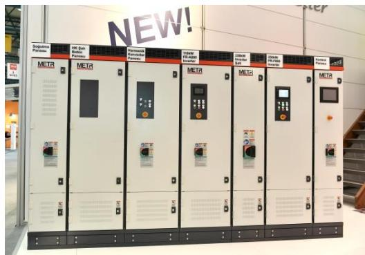
Mitsubishi Electric's new platform boasts of a modular design equipped with bar systems and accessories meeting EN 61439-1/2 type test standards and manufactured in line with assembly instructions in addition to undergoing short circuit and temperature rise tests. Developed in line with Mitsubishi Electric's high quality principle, the platform
