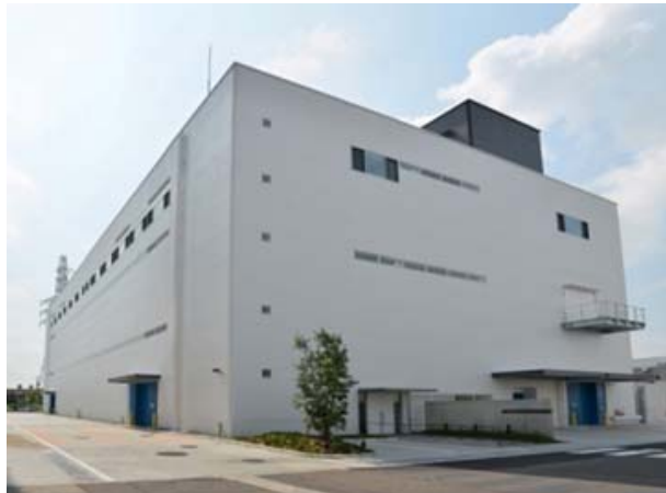
Elevators and Escalators QM center
