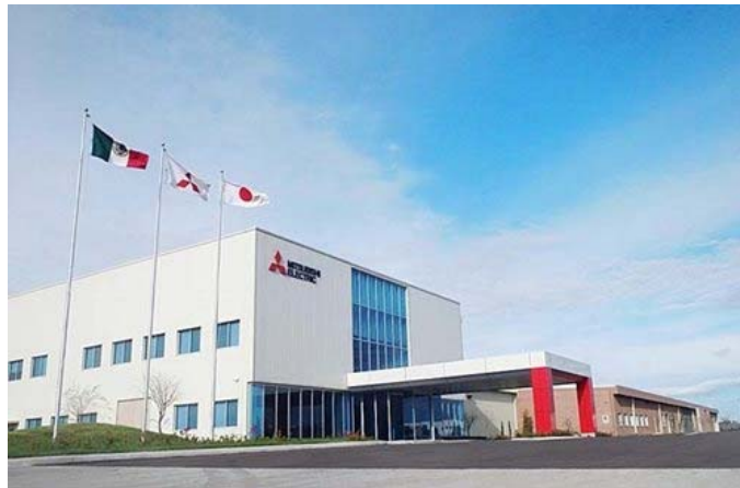
Business Centre where Mitsubishi Electric (Russia) LLC is located
